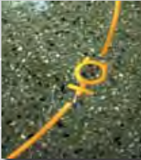
close-up of solar system
